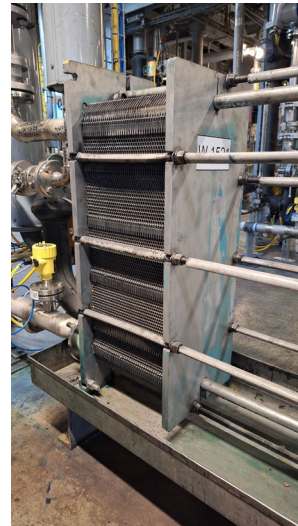
Plate heat exchanger
